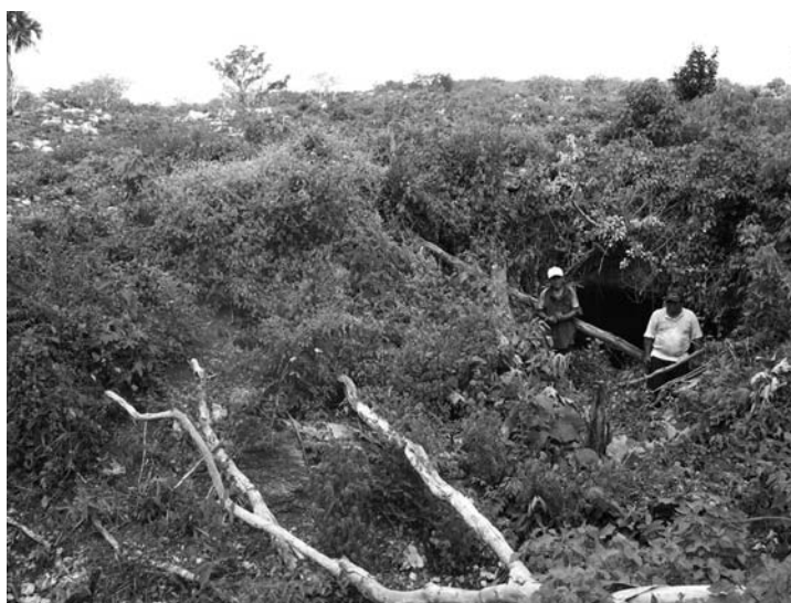
Figure 6. Collapsed saskabera along the Ichnul-San Andres causeway.
