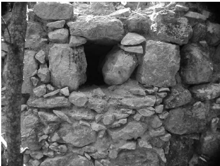
Figure 34. Exterior wall of the top level of S1E1-1.
