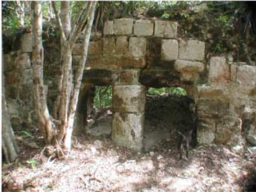
Figures 8a and 8b. Photographs of Structures N8W1-3 (top) and N8W1-9 (bottom)
