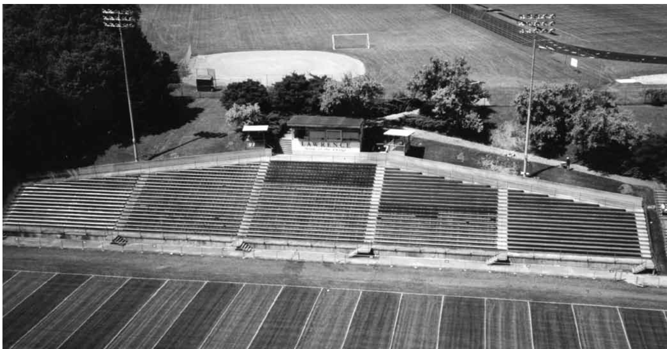
The Banta Bowl, constructed in 1965, is regarded as one of the finest small college football stadiums in the country.
