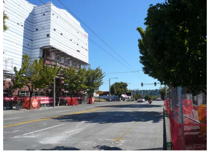
Figure 5 • View B, viewing east towards NW Market Street from 17th Avenue NW
