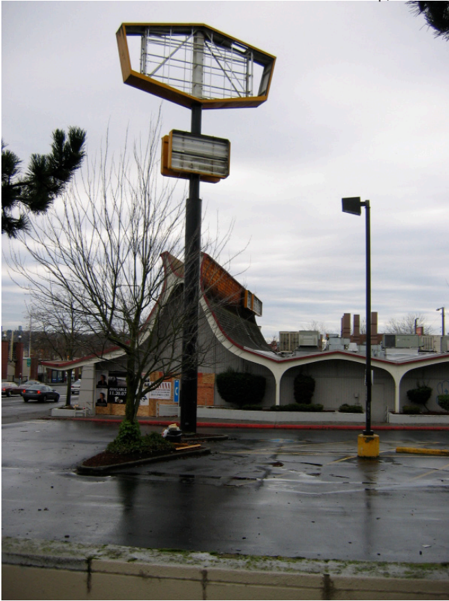
Figure 69 • Ballard Denny's, signage and north side, November 16, 2007
