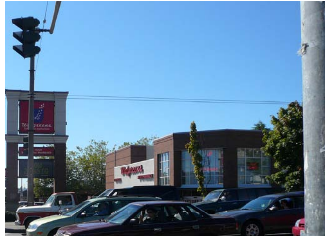
Figure 7 • View D, viewing south toward Walgreens from corner of NW Market Street and 15th Avenue NW
