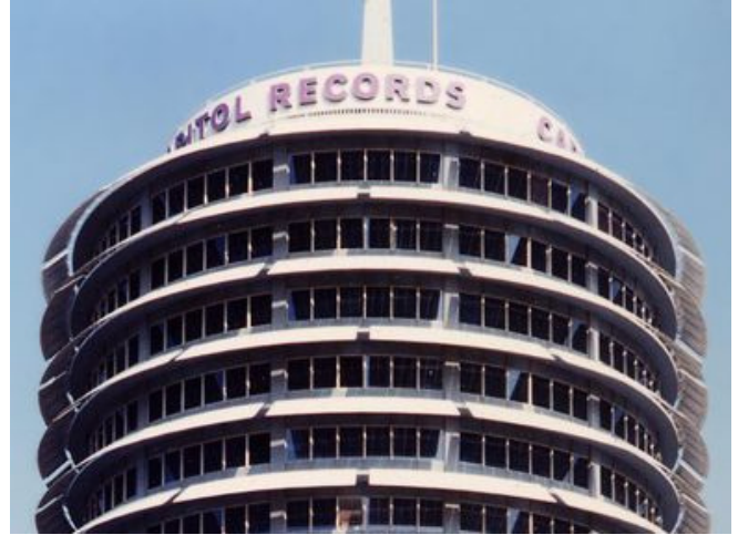
Figure 60 • Capitol Records Building, Hollywood California, 1956, Welton Beckett
