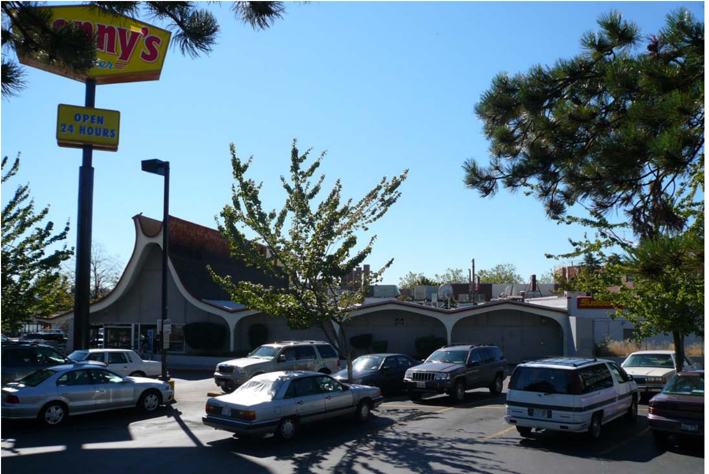
Figure 16 • North side and parking
