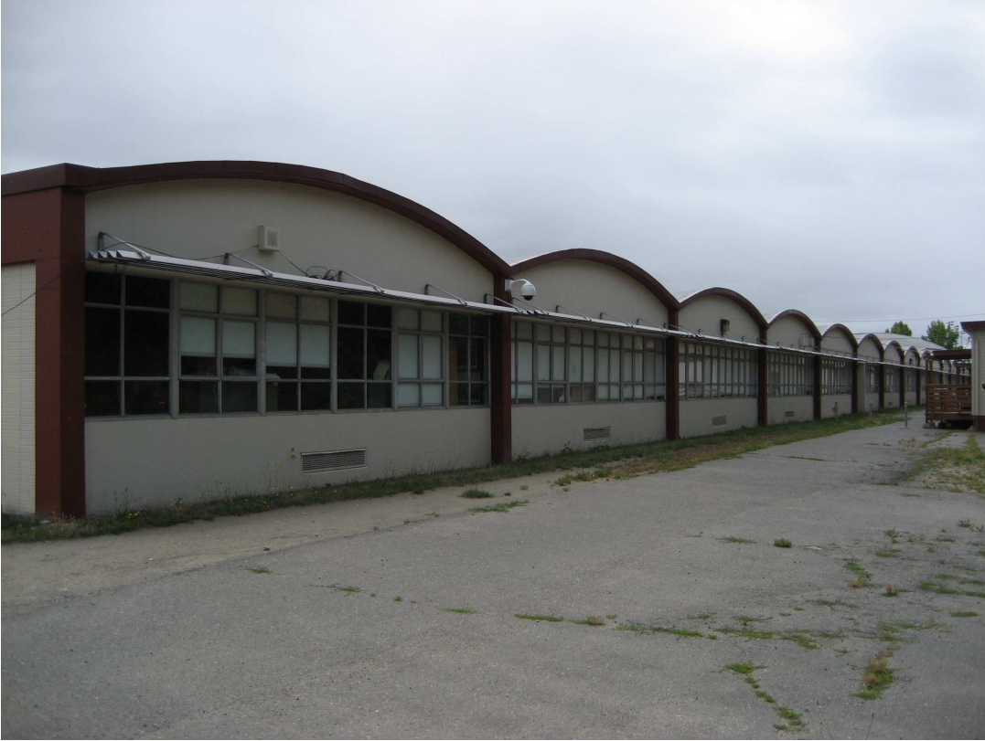
Chief Sealth High School Photo 11 – Main Building looking Southeast (2007)
