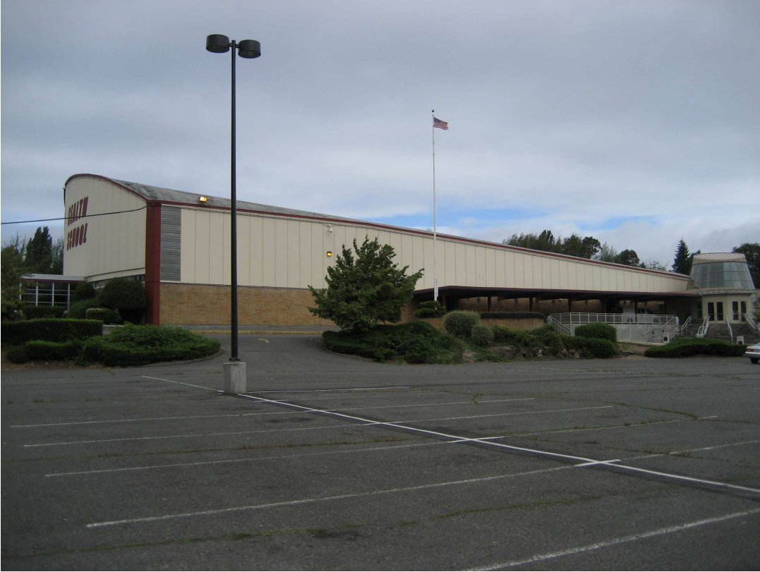
Chief Sealth High School Photo 3 – Auditorium looking West (2007)
