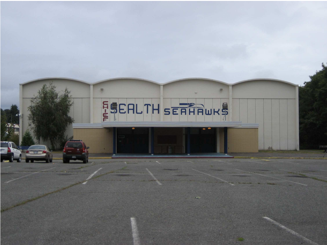
Chief Sealth High School Photo 4 – Gymnasium looking North (2007)
