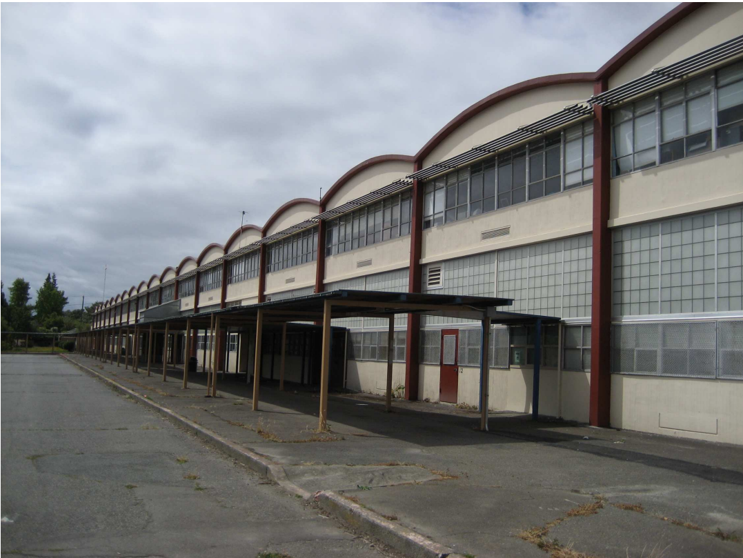
Chief Sealth High School Photo 10 – Main Building & Covered Walkway looking Southwest (2007)
