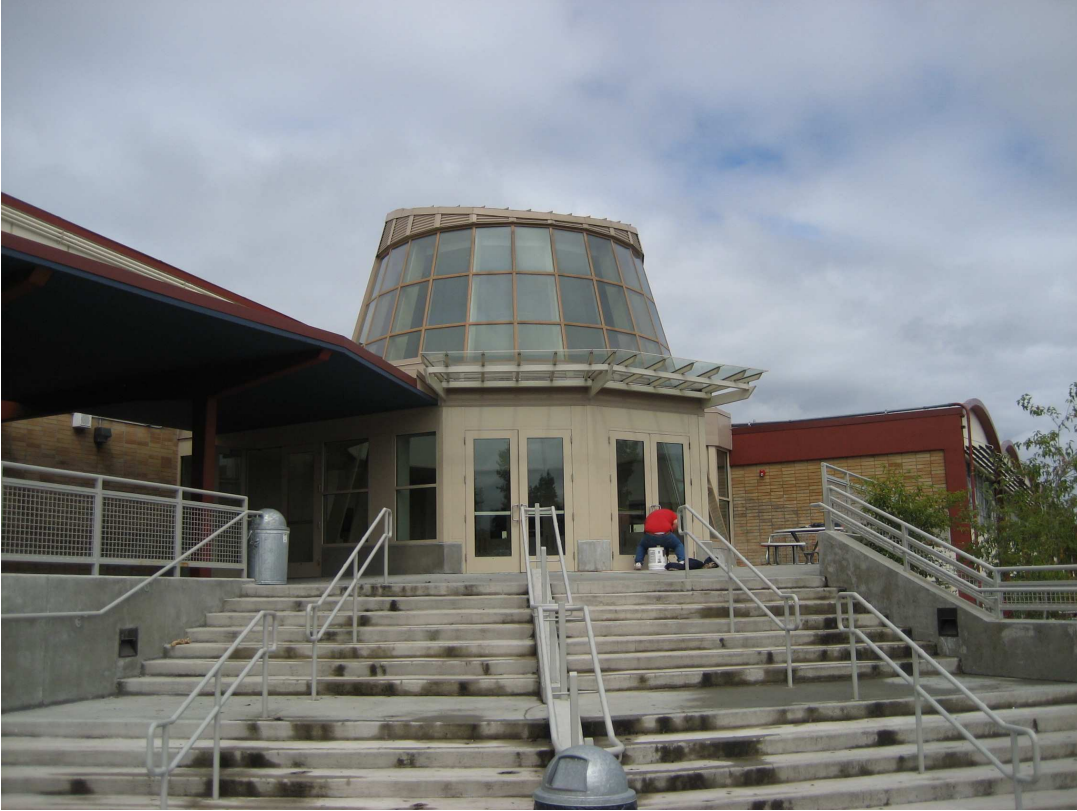
Chief Sealth High School Photo 7 – Main Entrance looking Northwest (2007)
