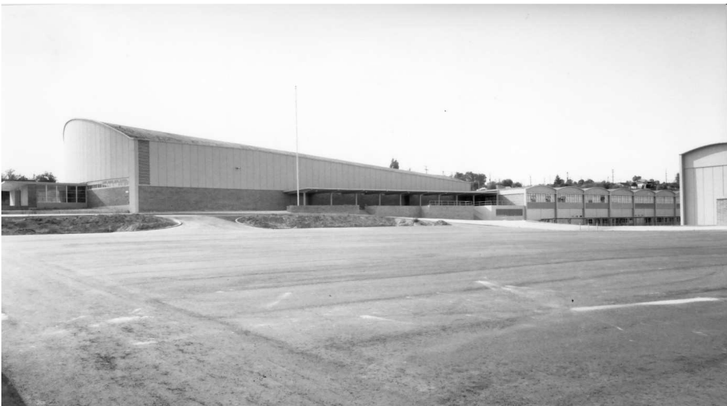
Chief Sealth High School Photo 2 – Auditorium looking West (1958)
