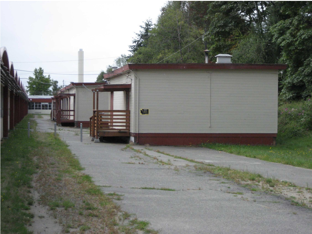
Chief Sealth High School Photo 12 – Portables (2007)
