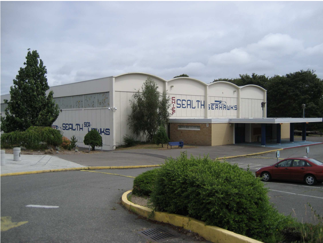
Chief Sealth High School Photo 8 – Gymnasium looking Northeast (2007)
