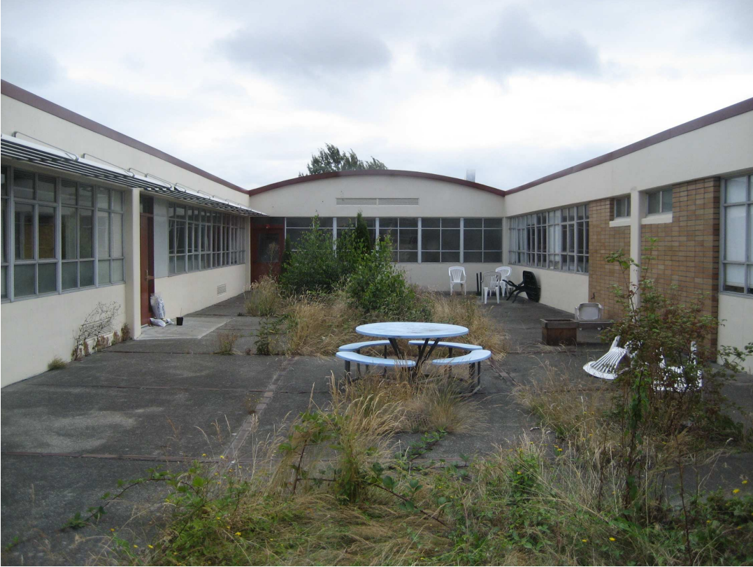
Chief Sealth High School Photo 15 – Exterior Courtyard (2007)
