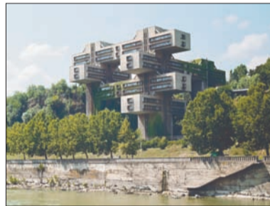
The Georgian Ministry of Highways in Tbilisi, built in 1974.
