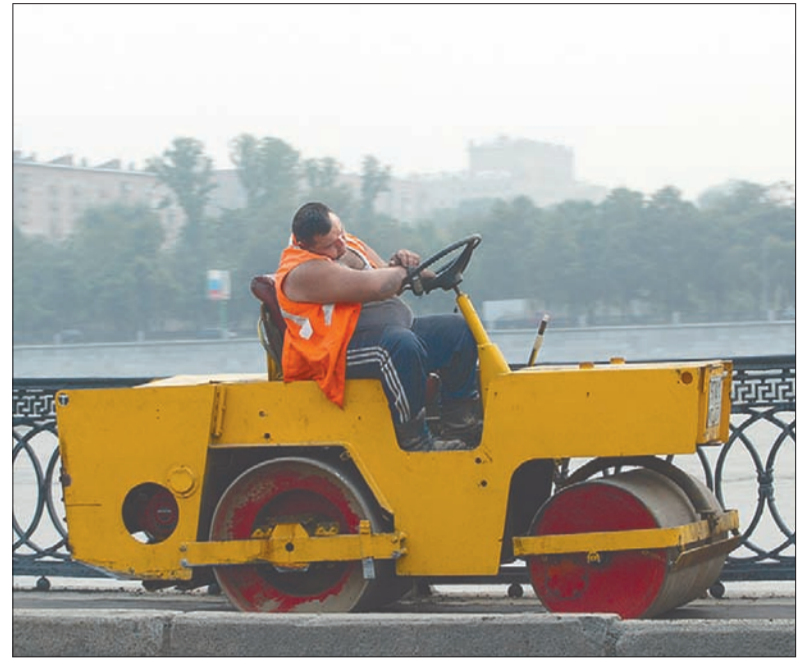
Very little funding has been allocated to road maintenance in recent years.
