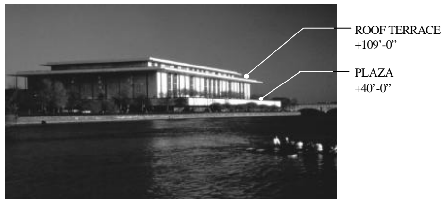
Figure 1: Overall view of the Kennedy Center looking from the northwest
