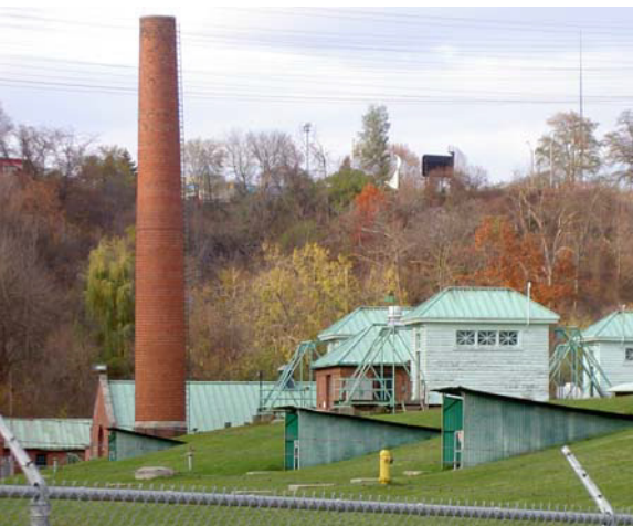
The North Toronto Sewage Treatment Plant is located at the centre of Crothers' Woods.
