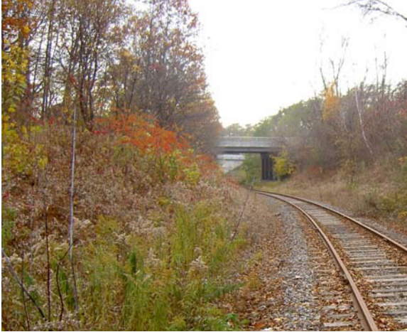
Rail lines border the site on the west and east.
