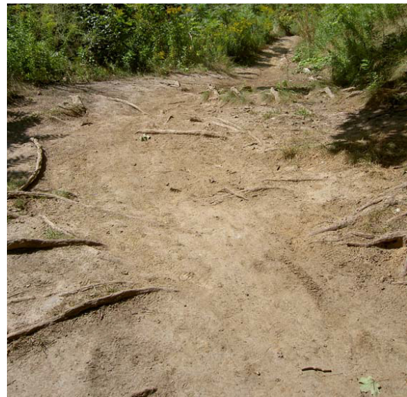
Soil erosion from improper trail design.
