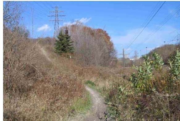
Natural surface trail along steep slope within old field habitat (CUM1-1) of hydro corridor, north of Pottery Road, showing wheel rutting and pooling of water in a transverse drainage swale in immediate foreground. Fall line trail acts as conduit for sediments to a drainage feature.
