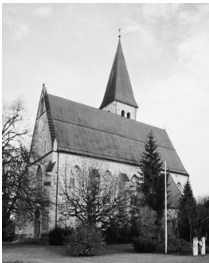
Parish church at Ruggell (left) and the «Biedermann House» at Schellenberg (right)
