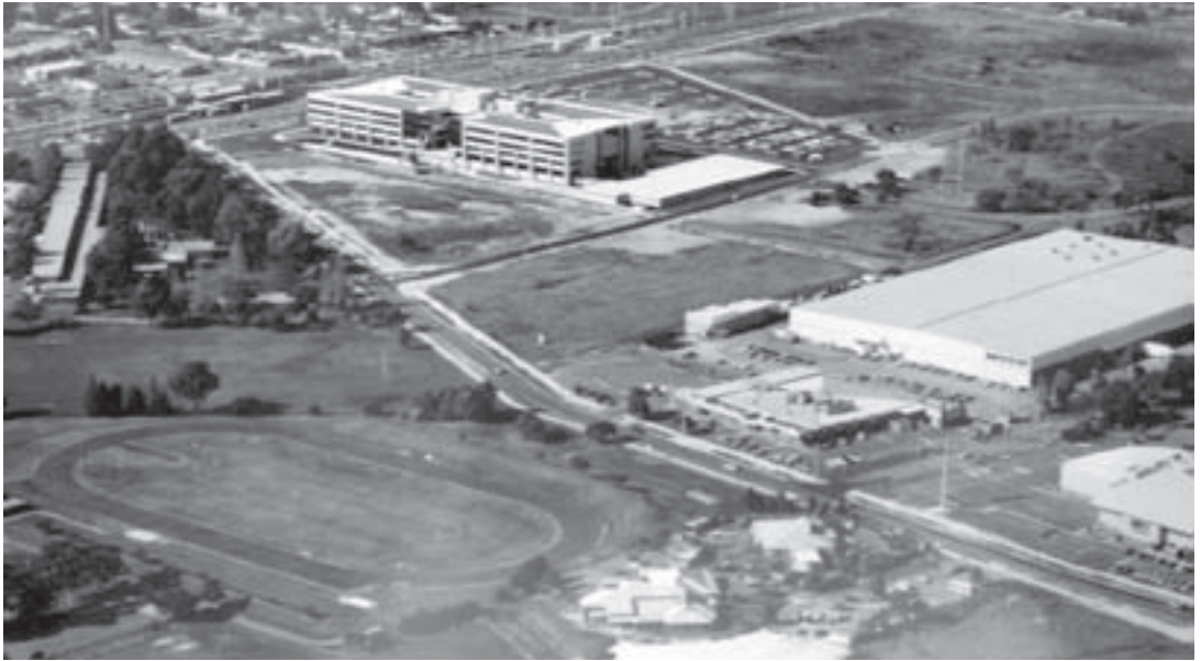
Cannington office in suburban Perth.
