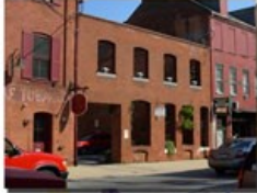
Preserved building facade serves as a gateway element
