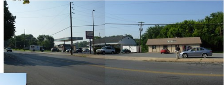
Low, suburban-style commercial development at Hershey Avenue is primarily designed for motorists rather than pedestrians from surrounding neighborhoods
