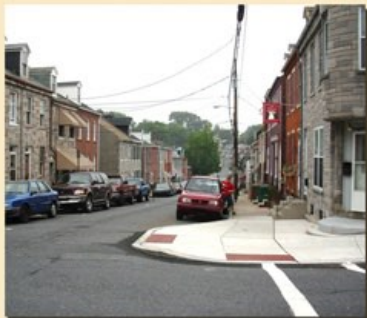
Recently installed curb extension, accessible ramps, and crosswalk.
