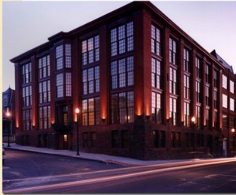
Example of facade lighting for landmark structures (Image Courtesy of Brinjac Engineering)
