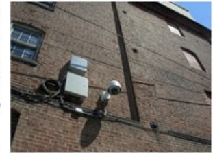
Existing surveillance camera located at South Water Street
