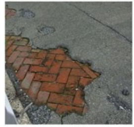
Remnants of earlier porous paving can be seen through later impervious pavement overlays
