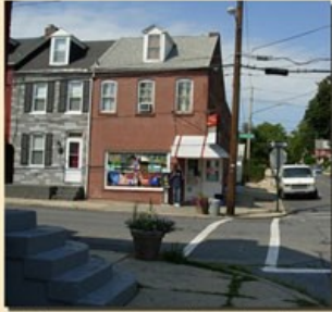
Existing corner store serving southwest neighborhoods
