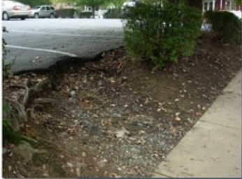
With topographical modifications, areas such as this eroded space adjacent to a Lafayette Street parking lot could serve as a storm water infiltration area
