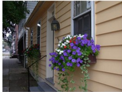
Existing front stoop lighting on West King Street
