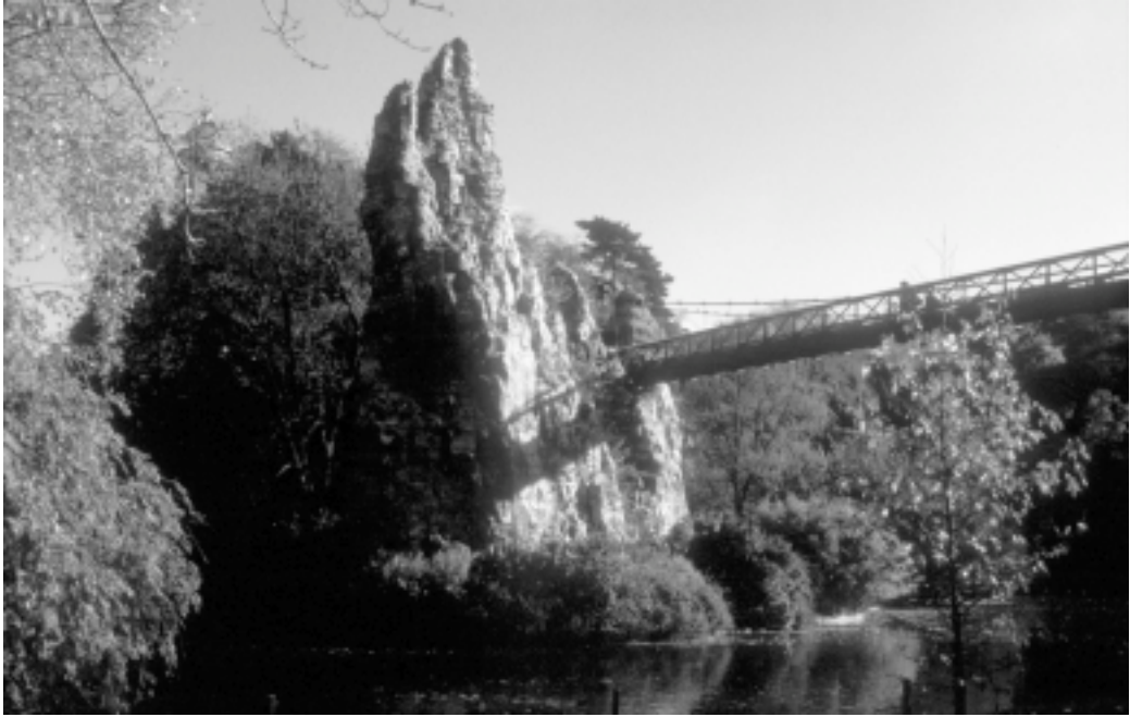
12. Steel-cable suspension bridge, Buttes-Chaumont, 1997
