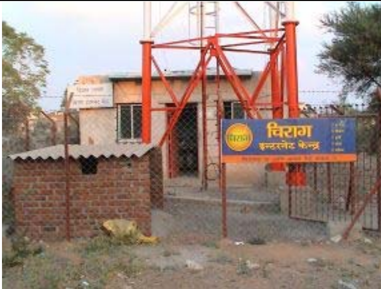
Below: Nlogue Access Center at Rajgurunagar
