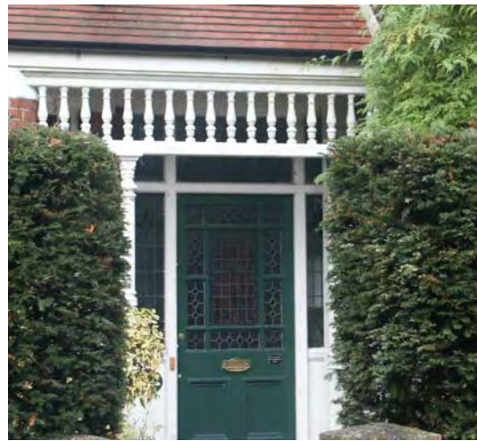
Dryden Road: porch
