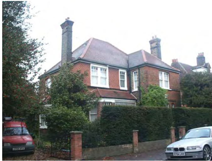
Dryden Road: 1 st phase house
