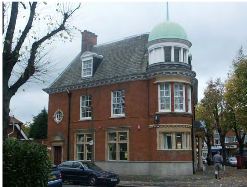
Former bank building
