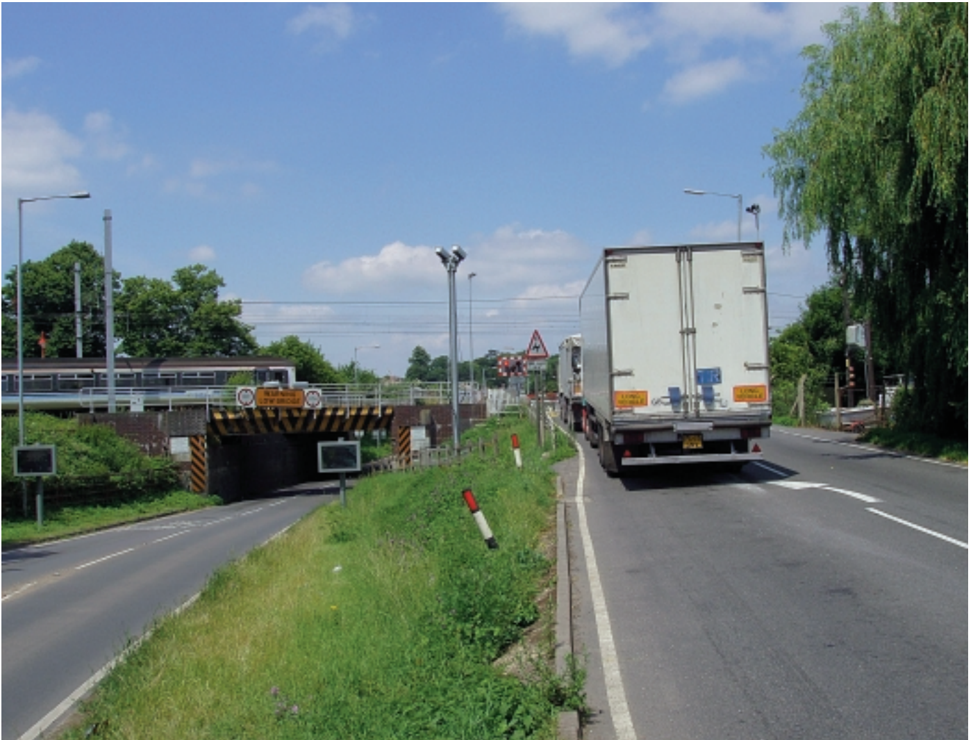
Level crossing at Ely
