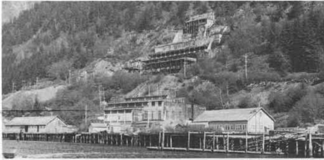
The ruins of the Alaska-Juneau mill hang above the southeastern end of Juneau. (R) Lower Salmon Creek powerhouse: 2500-HP impulse turbine by the Pelton Water Wheel Co. (San
