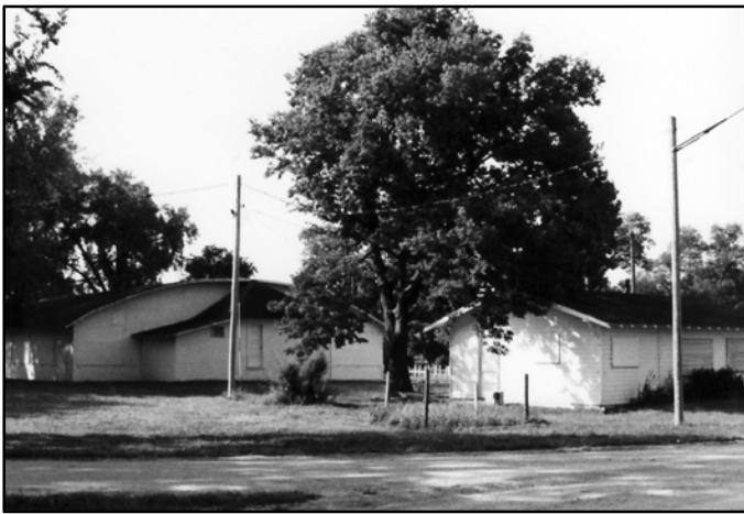
Photo 1 of 5 – dance pavilion & restroom/concession bldg, looking SW Photo by Carol Ahlgren, 1998, NSHS (9808/3:4)
