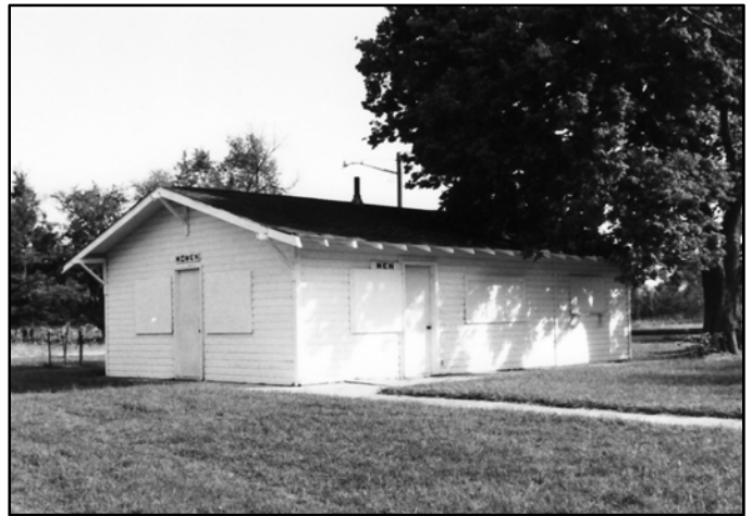
Photo 2 of 5 – restroom/concession bldg, looking NE Photo by Carol Ahlgren, 1998, NSHS (9808/3:1)
