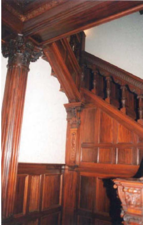
Staircase to third floor
