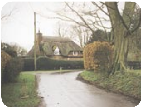
Church Cottage from the west
