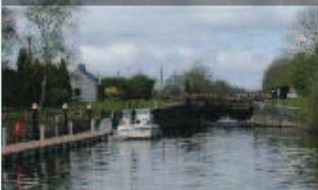
Approaching Albert Lock Photo: Richard Ellis
