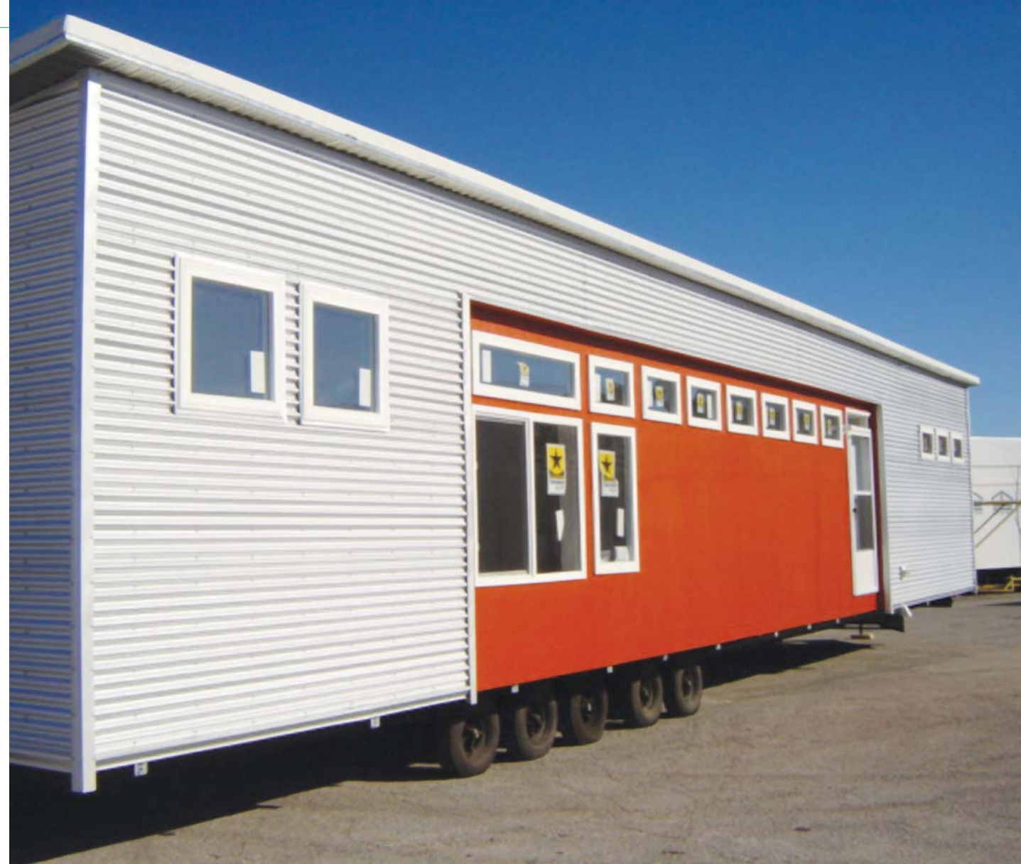
Above Delivery of the manufactured unit. 2008
