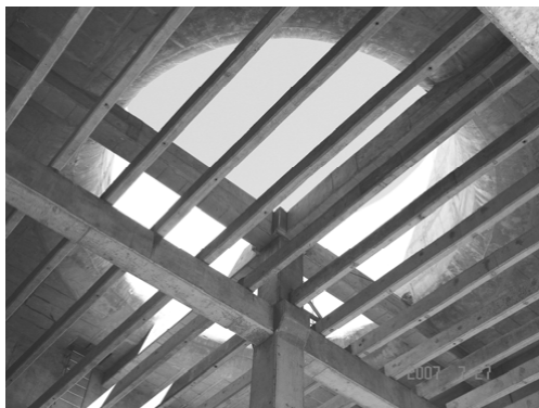
Figure 8. Civil construction inside cooling tower
