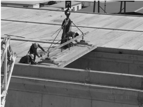
Figure 5. Pre-cast roof slabs of air cooler.
