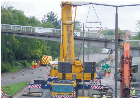
● Demolition of St Alkmund's Way footbridge
