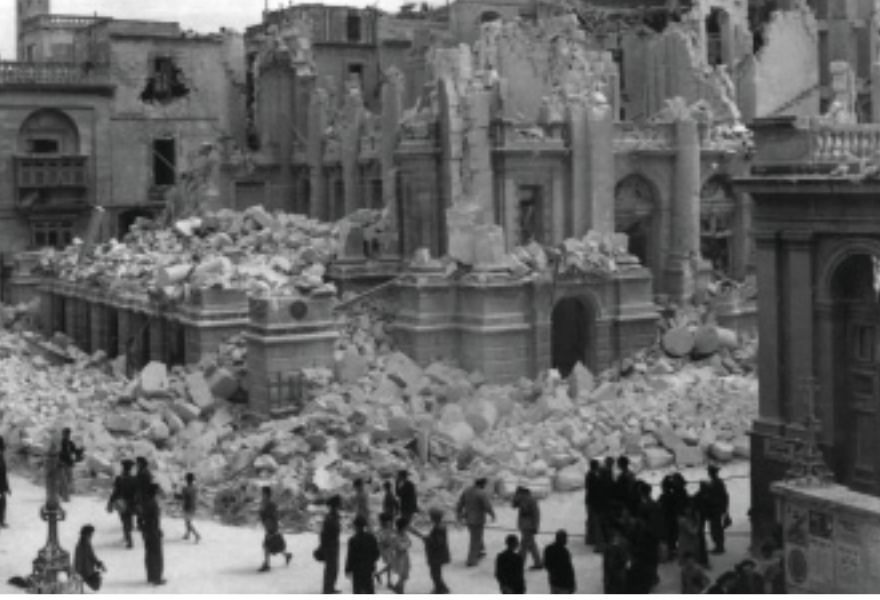
Valletta Opera House, Malta, destroyed
