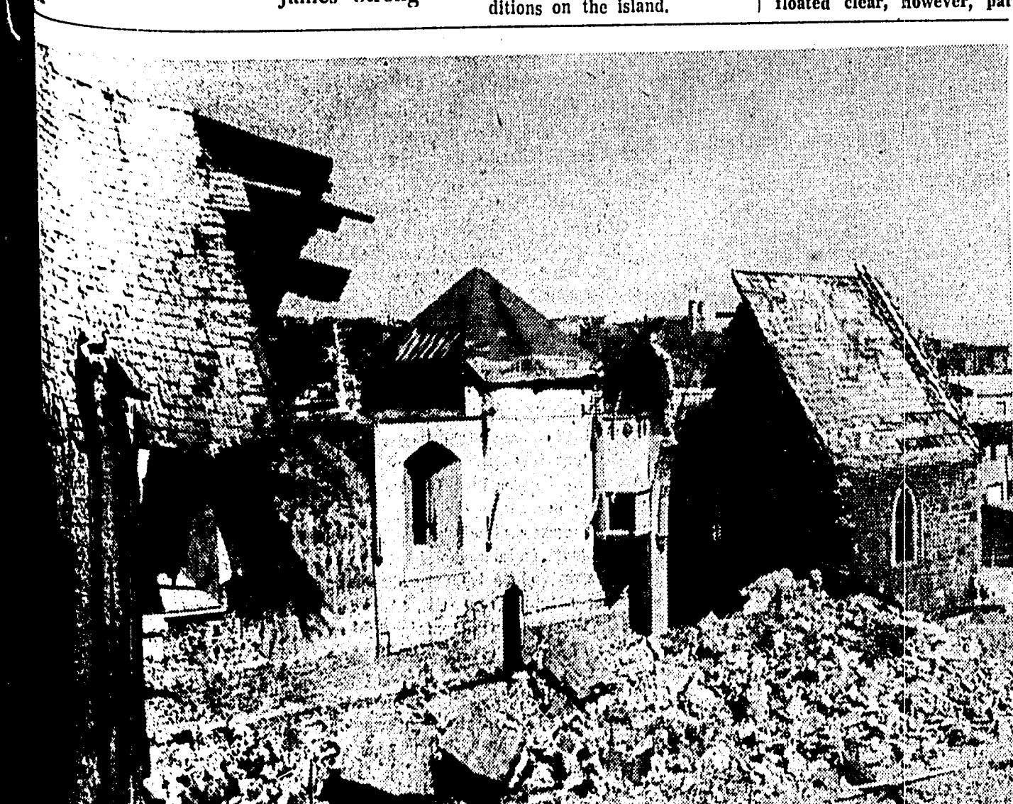
BEING DESTROYED—The old St. Mary's Church, a landmark on the South Side of St. John's, is now being destroyed as a way for the final phases of the harbor development. The 103 year old building was vacated in 1962 when a new church was opened on Craigmillar Avenue. The church is seen after 30 charges of dynamite had been set off in it.—(News Photo)
