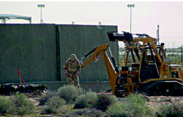
A sandbag bunker and concrete revetments provided additional protection from the bomblet's fragmentation.
