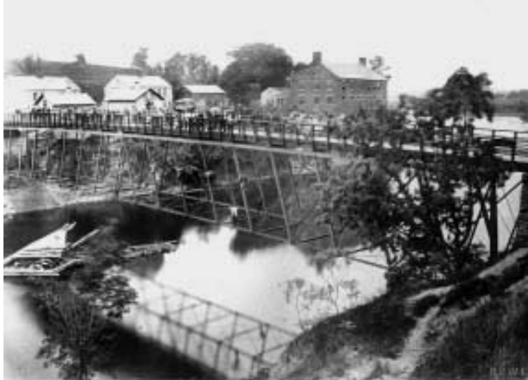
STOCKPORT BRIDGE, COLUMBIA, CO. N. Y. SPAN 343 FEET
