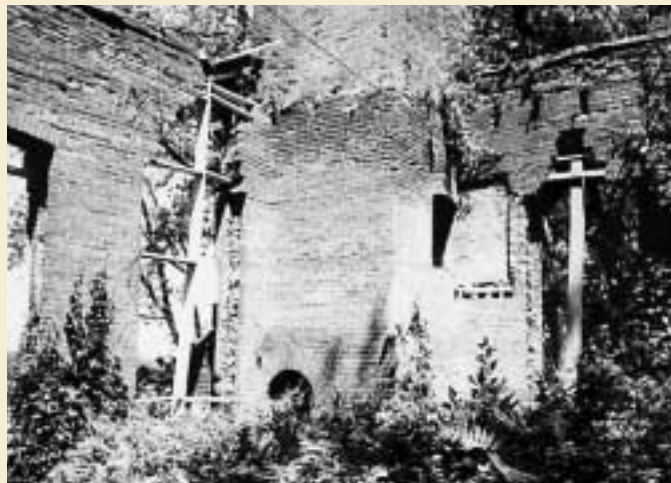
North west view of interior of the Power House.
