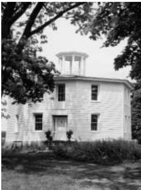
Front view of Johnathan Hallam's restored home with rooftop cupola from which majestic views may again be enjoyed.
