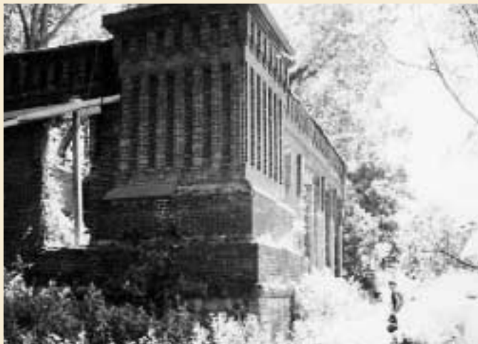
Remains of the Brick Power House.
