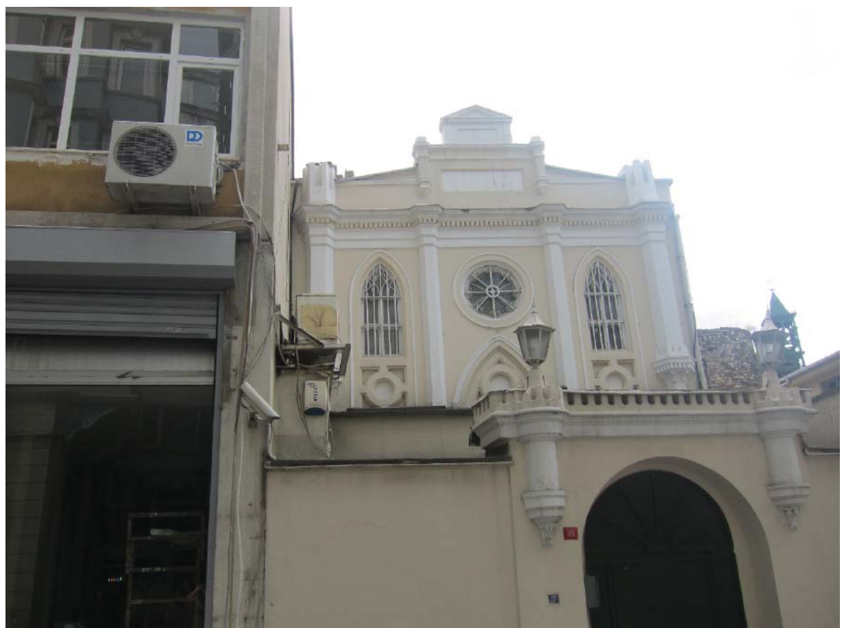
Exterior of the Italian synagogue in Istanbul. Note the thick concrete wall, thick steel doors and cameras overlooking the street
