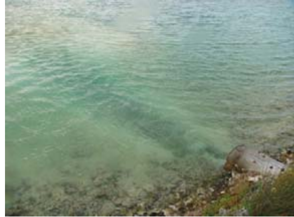
Figure 4.17: Seawater outlet at Site "5"
