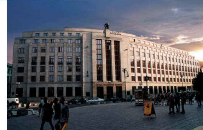
The current headquarters of the Czech National Bank and its Prague branch in Na Příkopě St.
