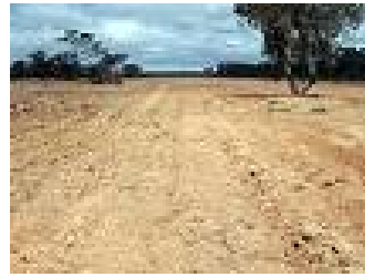
The same excavation infilled and prior to revegetation
