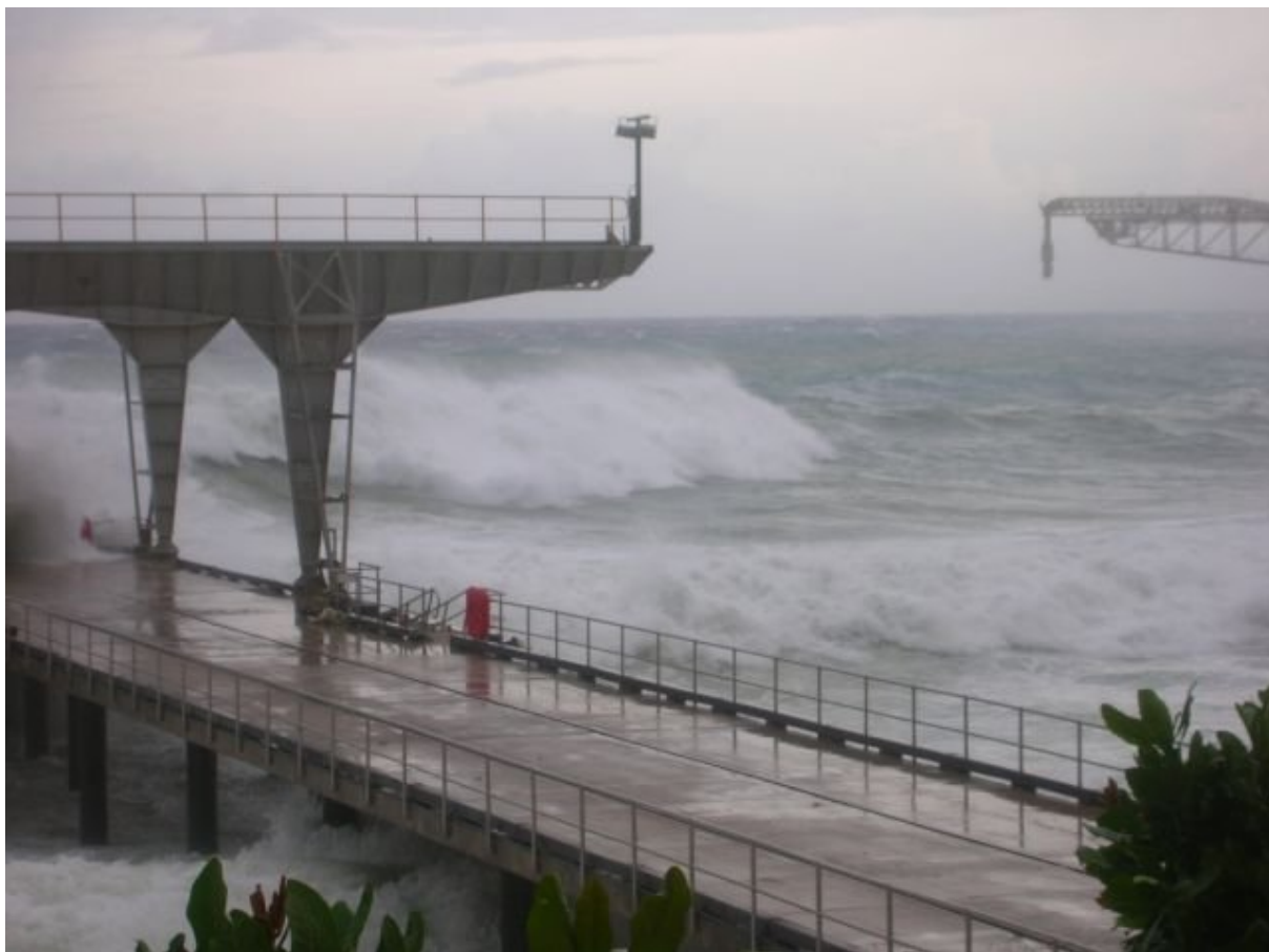
Figure 7.3 Large waves at the Christmas Island Port. Photo provided by Dave Robertson, Harbourmaster, Christmas Island Port.
