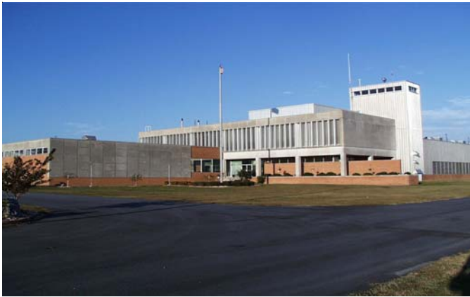
Figure 1: Site A, Greenville Transmitting Station
