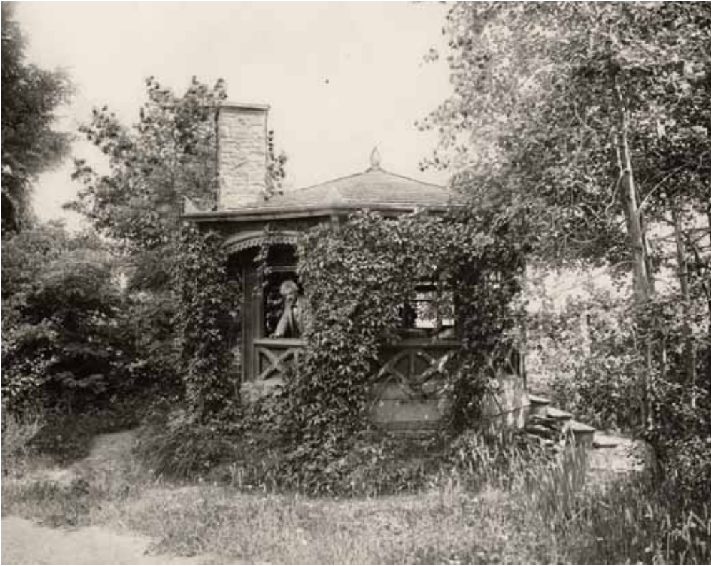
Samuel Clemens looks out the window of the octagonal study that Susan Crane built for him up the hill from Quarry Farm.
