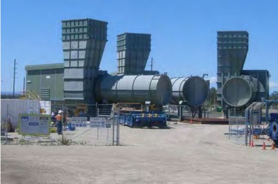
Plate 2-4 Blakefield South No 2 ventilation fans under construction
