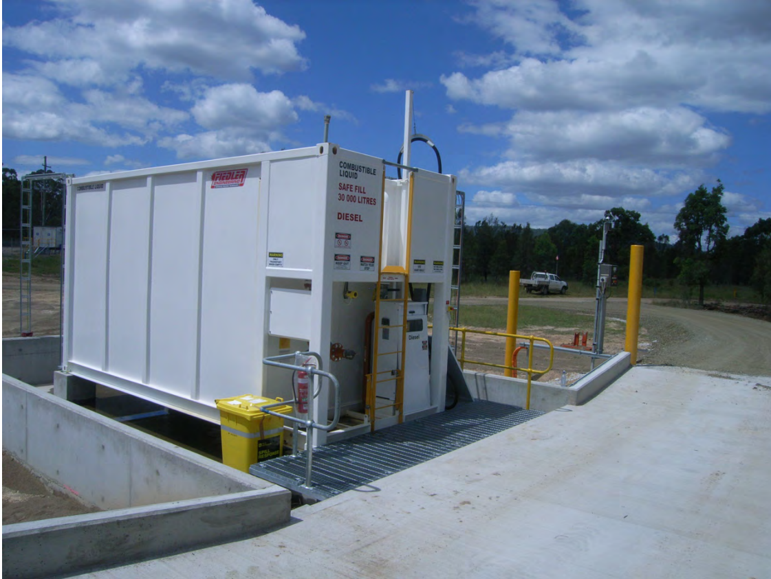
Plate 2-1 The gas drainage hydrocarbon storage facility constructed during the reporting period
