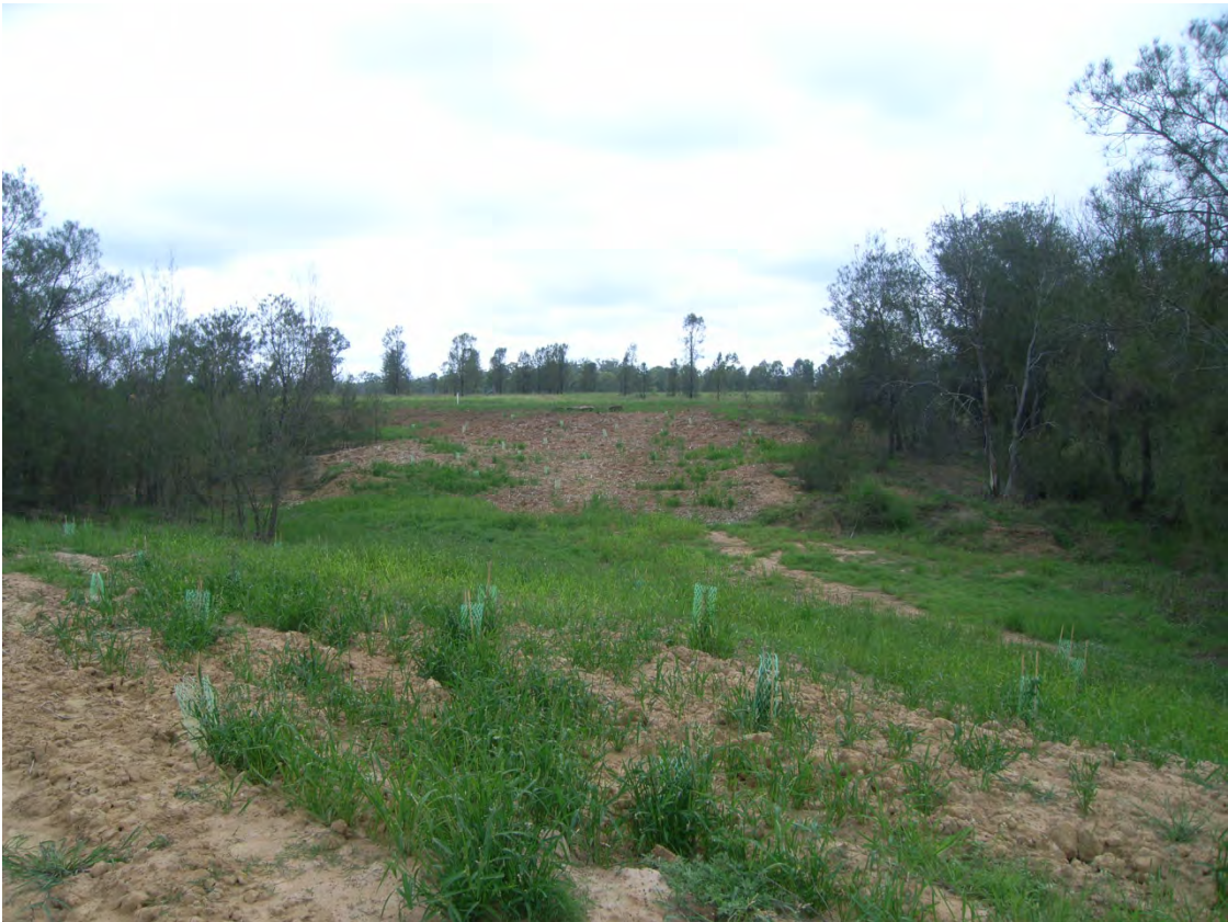
Plate 2-14 The same slope along the Northern Drainage Line 3 months after rehabilitation
