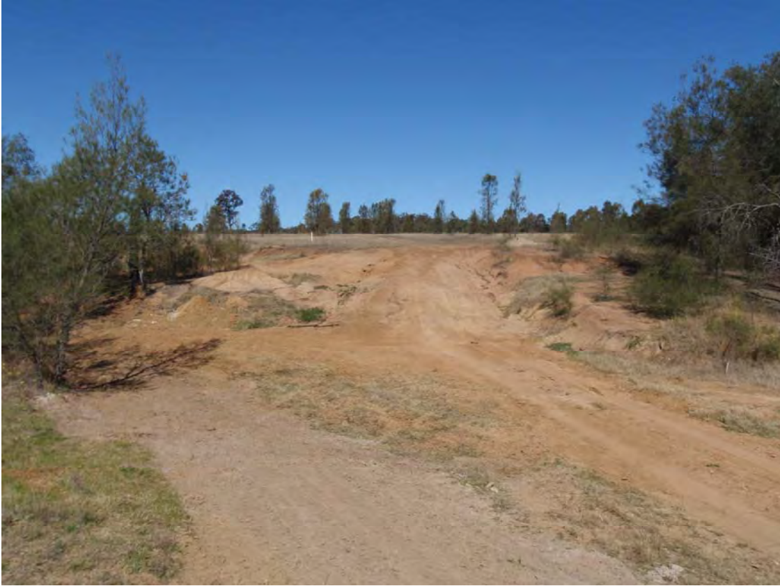
Plate 2-13 A bare eroded slope along the Northern Drainage Line prior to rehabilitation
