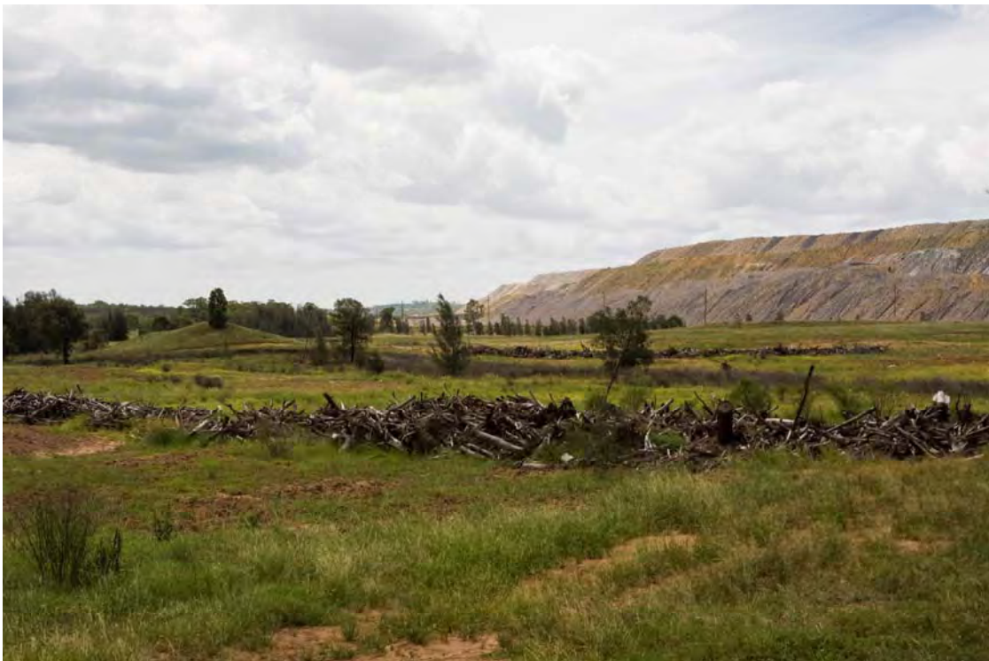
Plate 2-12 Rehabilitation works on the Northern Drainage Line over Longwall 9 following December rainfall
