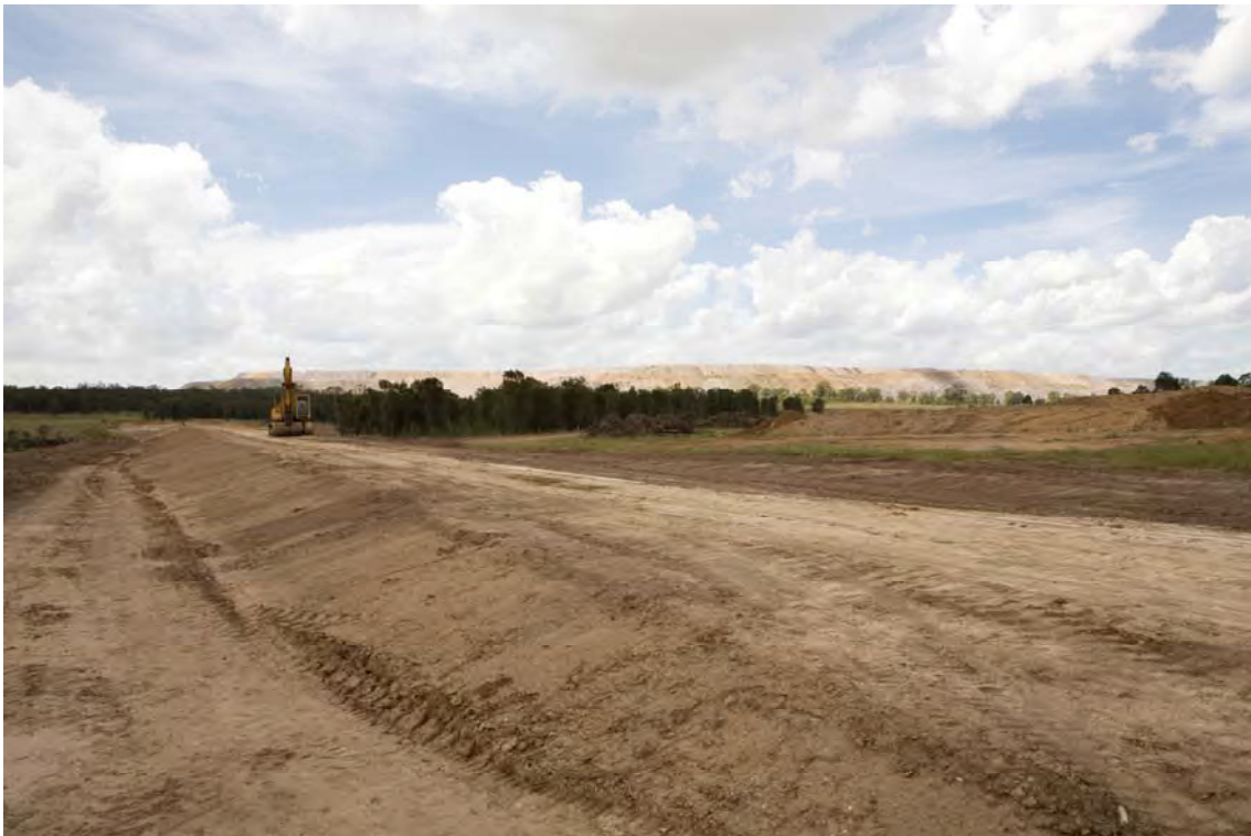
Plate 2-3 The Wollombi Brook Flood Levee as commenced in December 2009
