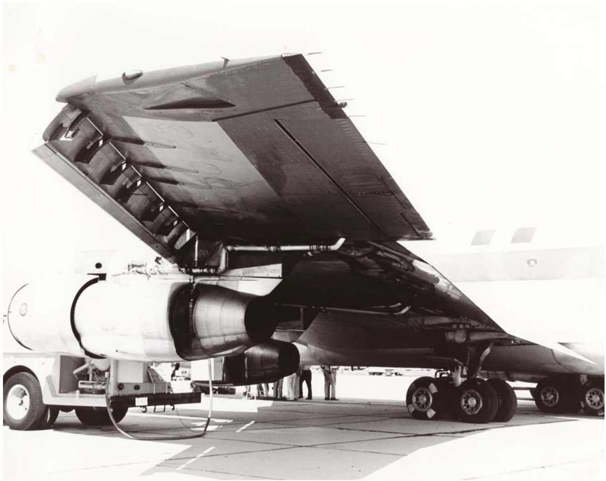
This series of seven photographs by G. Harry Stine shows the original Boeing 387-80 prototype of the 707 airliner on the ramp at NASA Wallops Station, Virginia, in June 1964 . The “Dash 80” had been modified for very slow flight using wing flaps blown by Coanda Effect. Primary air for blowing the flaps came from compressor bleed of the Number One and Number Four engines. Aircraft could fly as slow as 70 knots. (70 knots = 80.6 mph = 129.85 kph which is about half its normal takeoff speed)
