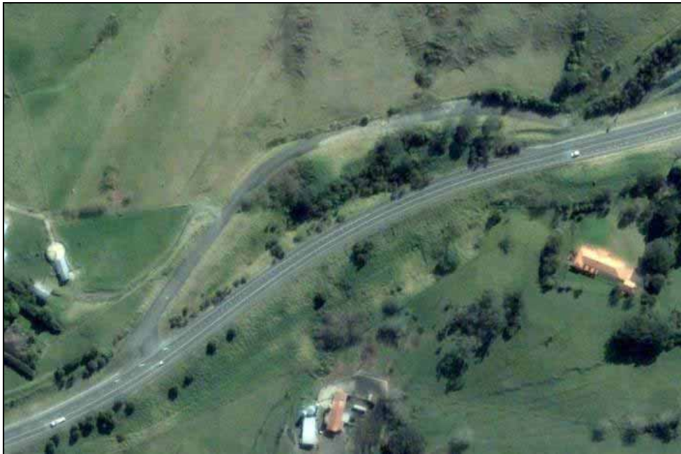
Figure 8.58: Aerial view of highway remnant G2B H33 (Google Earth image 2010)
