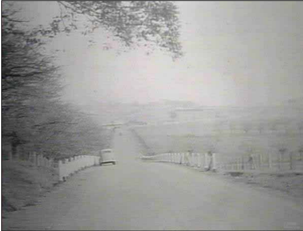
Figure 7.15: View looking southwards along the new 'Omega Deviation' (Gerringong Bypass), State Highway 1, from front of Renfrew Park , Sep 1938
