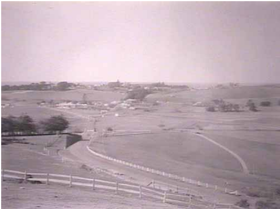
Figure 7.18: View of the southern end of the Gerringong Bypass completed in 1936, looking east. This section of the bypass cut off a number of bends, shown in the 1920s view, Figure 7.14.
