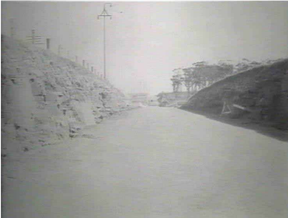
Figure 7.17: View of rock cuttings along the 'Omega Deviation', in 1938 looking south-west
