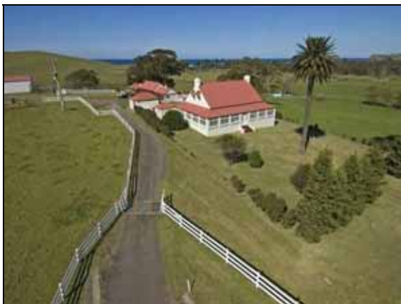
Figure 8.81: G2B H38 – .Oblique aerial view of homestead and front grounds looking south-east. Note recently constructed driveway and entrance
