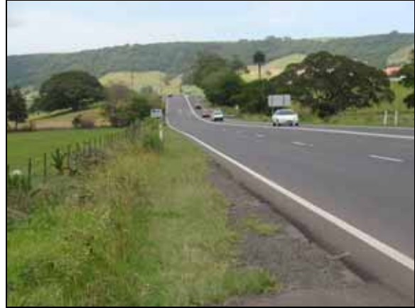
Figure 8.30: PASA 38 – view looking north from Omega Flat, towards spurline
