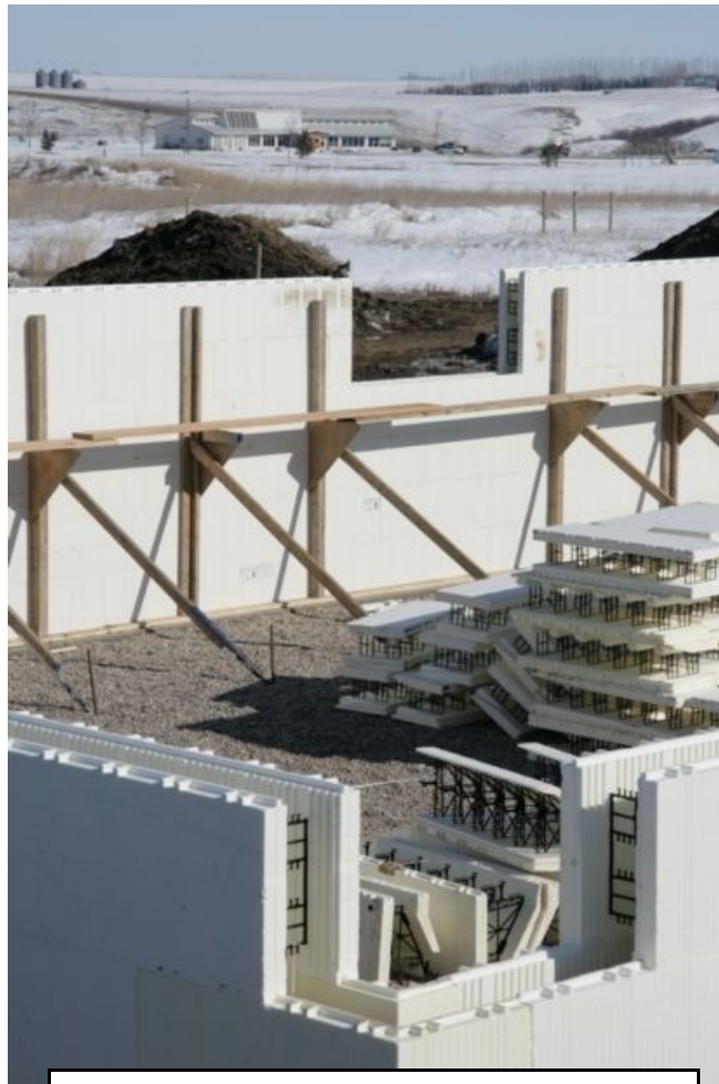
Praxis' insulated concrete forms being used at Craik Ecovillage.
