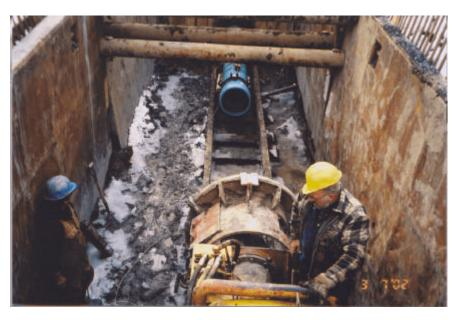
Consumers Gas, Toronto Hydro, Hydro One, Bell Canada, and TransNorthern Pipelines. LEA worked closely with Enbridge Consumers Gas to negotiate the lowering and relocation of a 400 mm dia. High Pressure Gas Main in Neilson Road. Numerous discussions and meetings were required with Bell and Toronto Hydro to negotiate the relocation of underground plant and pole
