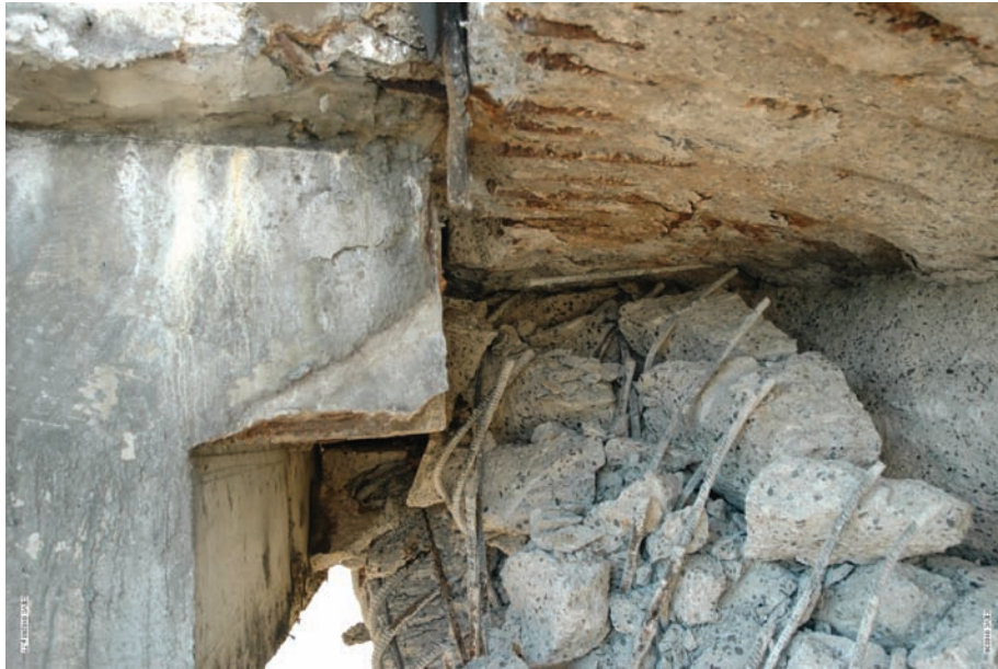
Figure 6.6 Photograph of the area of the corbel, towards the center of the abutment, where the slab stopped splitting. 8
