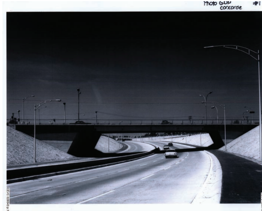
Figure 4.2 The de la Concorde overpass, north-bound
