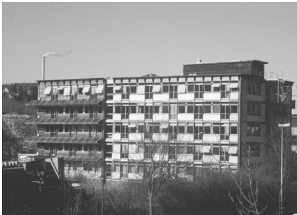
Figure 1b: East Façade
