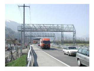
Furthermore, the Customs Administration checks that the HVF declaration is correct with fixed and mobile monitoring points in traffic. The data from the recording device is transmitted via the DSRC radio link by the current 23 fixed monitoring installations on the Swiss motorway network and is automatically compared with the data (number plate, vehicle length, etc.) captured electronically by the installation.
