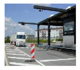
When the vehicle crosses the border the mileage counter is automatically switched on or off. This function is activated by a short-range microwave radio link using radio beacons installed above the road at the border crossing points, a type of radio technology called dedicated short-range communication (DSRC). DSRC has been standardised throughout Europe for electronic monitoring with a view to levying vehicle taxes.
