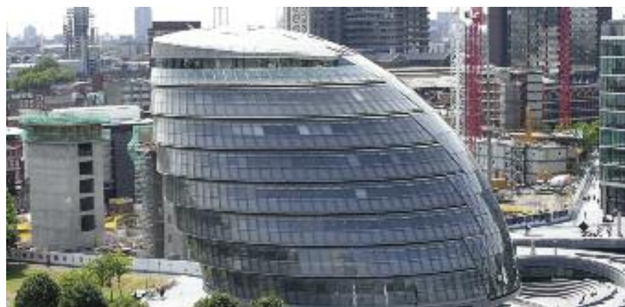
London city hall against a backdrop of construction activity.
