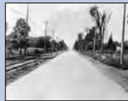
In 1909 Woodward Avenue became the country's first stretch of roadway paved with concrete.
