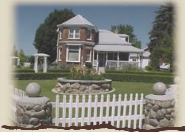
The heritage of the area is reflected in stately historic homes
