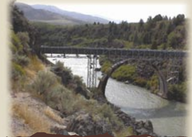
Last Chance Canal Flume, Bear River, near Grace, Idaho
