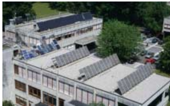
Figure 1: Test stand of the LEEE-TISO testing centre (left) and the TISO 10kWp grid-connected PV power plant (right).
