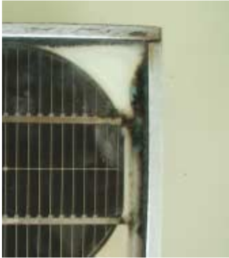
Figure 9: water penetration corresponding to the tedlar backsheet detachment in a 21-year old ASI16-2300 module.
