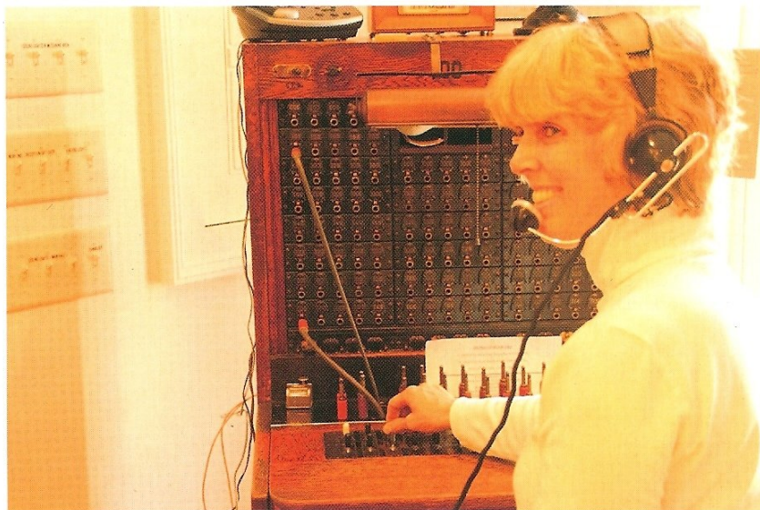
Always staying connected to her work, Carole Soule works the switchboard!
