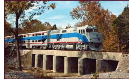
Bridge over Stoner's Creek
