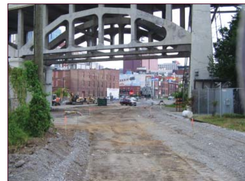
Riverfront Station Excavation 11-24-04
