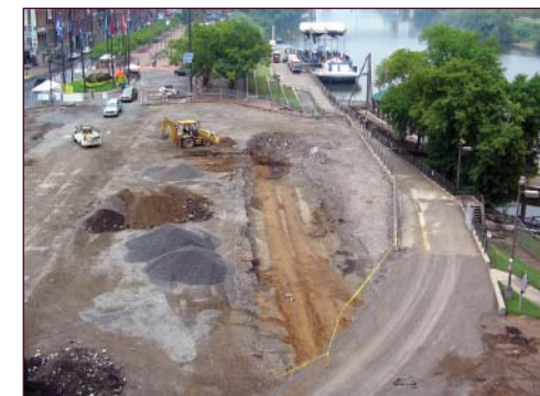
Riverfront Station Grading 8-25-05
