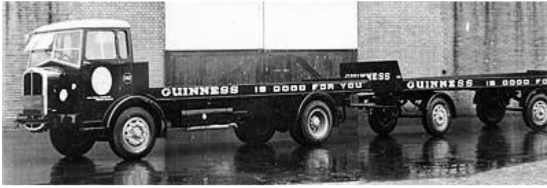
A bonnet extension indicates a six-cylinder engine for this forward-control Trusty.
